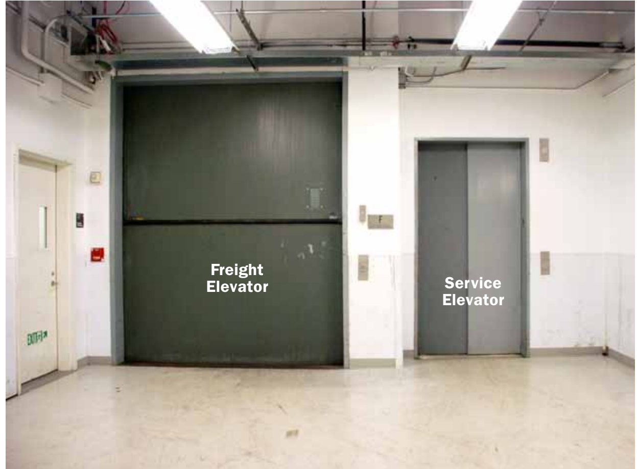
Freight and Service elevators on TimesCenter Hall level.
